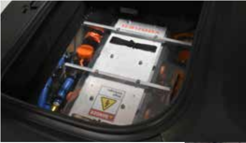
Batteries hidden in the boot
